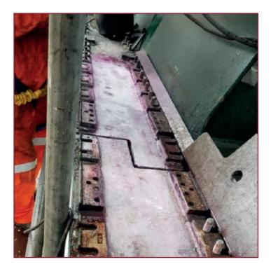
STARKON's rail sole plates are designed for long life, and only high-quality standard raw material is used during production. We can offer standard specifications AAS OEM requirements as well as improved sole plates. The function of sole plates is very important within systems of rail installation for overhead travelling cranes, harbour cranes or gantries.
